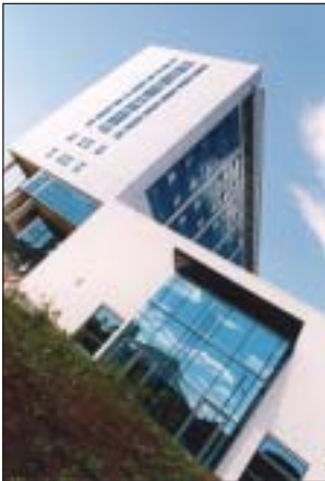
New Cardonald College Building
