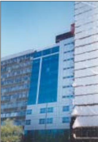
Cardonald College during recladding phase
